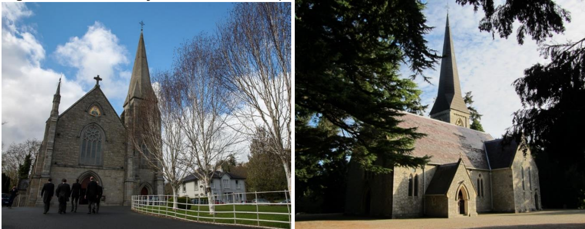
Figure 5.10 – St. Mary's Parish Church (left) and St. Patrick's Church (right)
